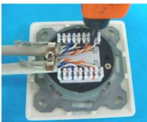
5. Adjust the gap on the cover to fit the cables. Latch the snag (the marked part in the following picture) to the hole on the body and then fasten the screw.
